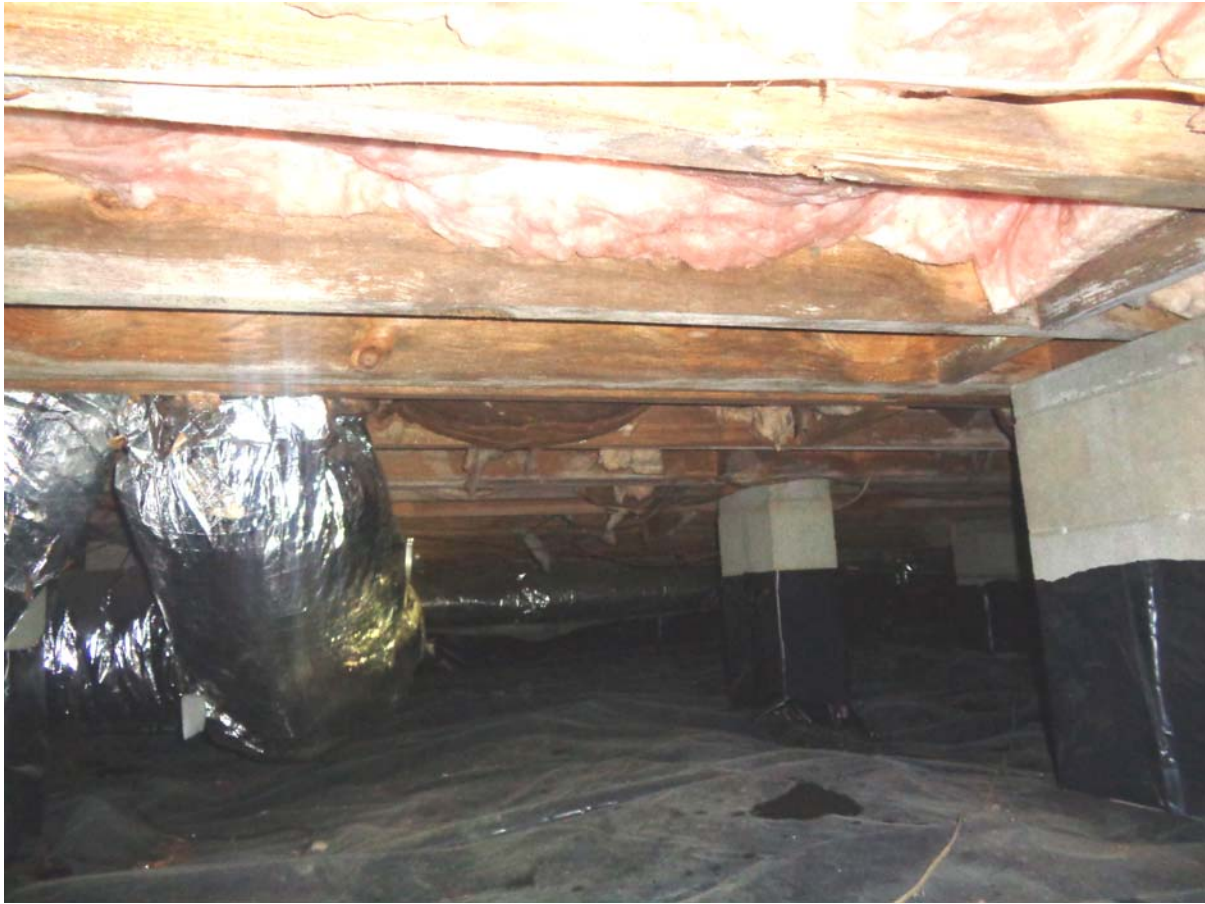
View of Crawl Space
